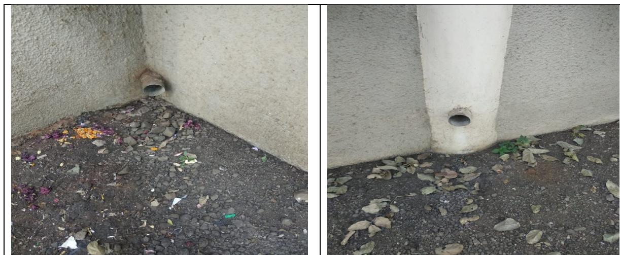
Fig 2. Rainwater harvesting system installed in the campus
